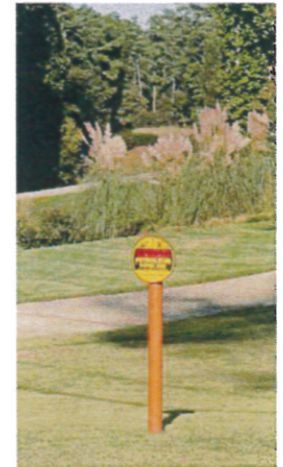
A pipeline marker is the only evidence of a pipeline buried underground.
